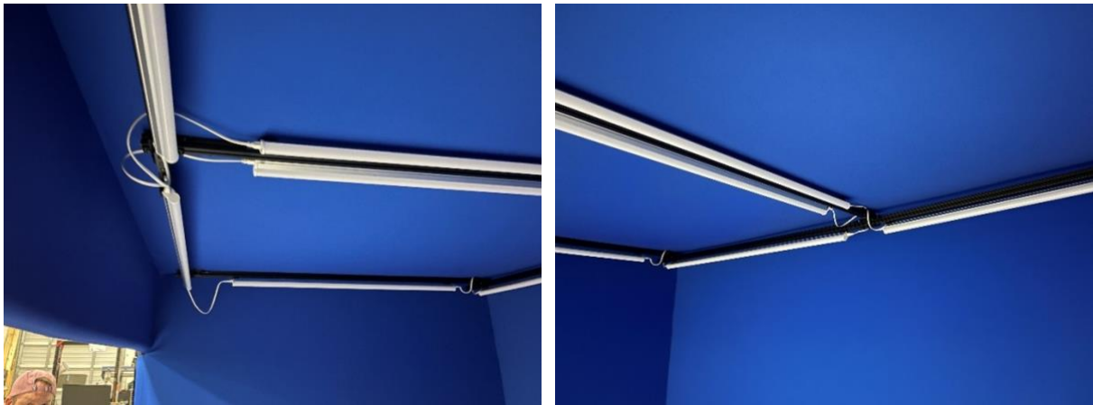
Figure 7-16. Connecting light to front wall
