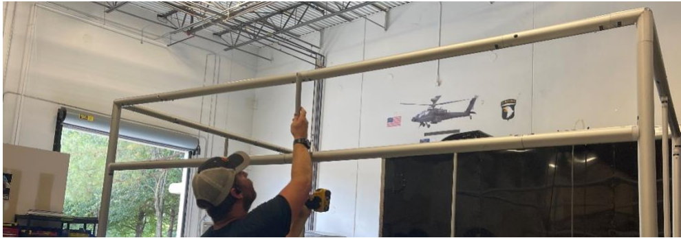
Figure 5-5. Securing the Silver Pipe
