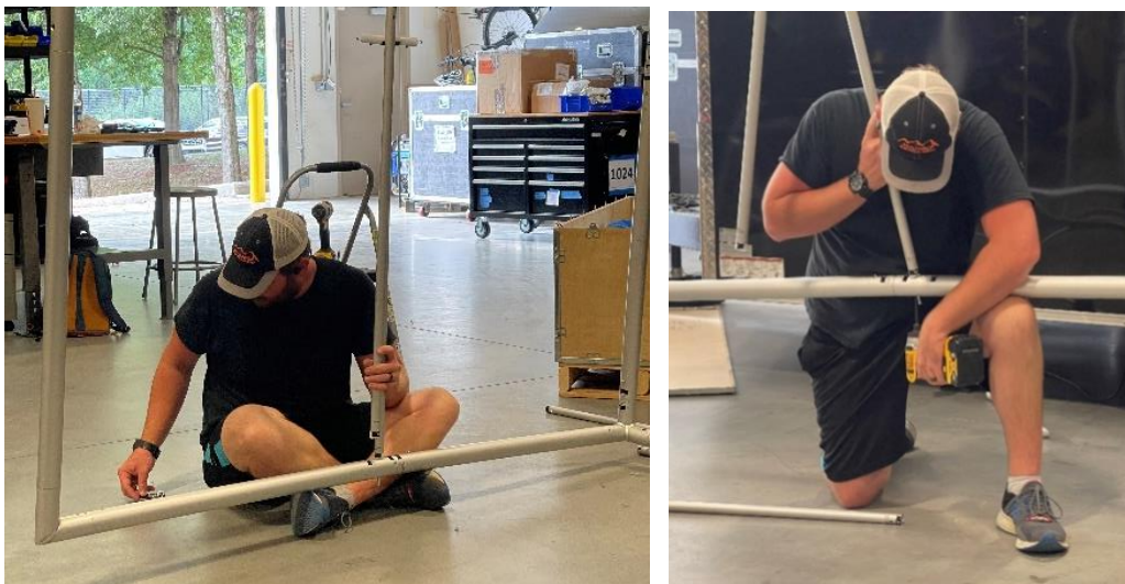
Figure 5-3. Installing Cross Member to its Bottom Pipe
